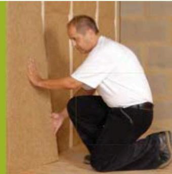
High carbon capture by Hemp fibre insulation fleeces. Picture: Hock (DE)
