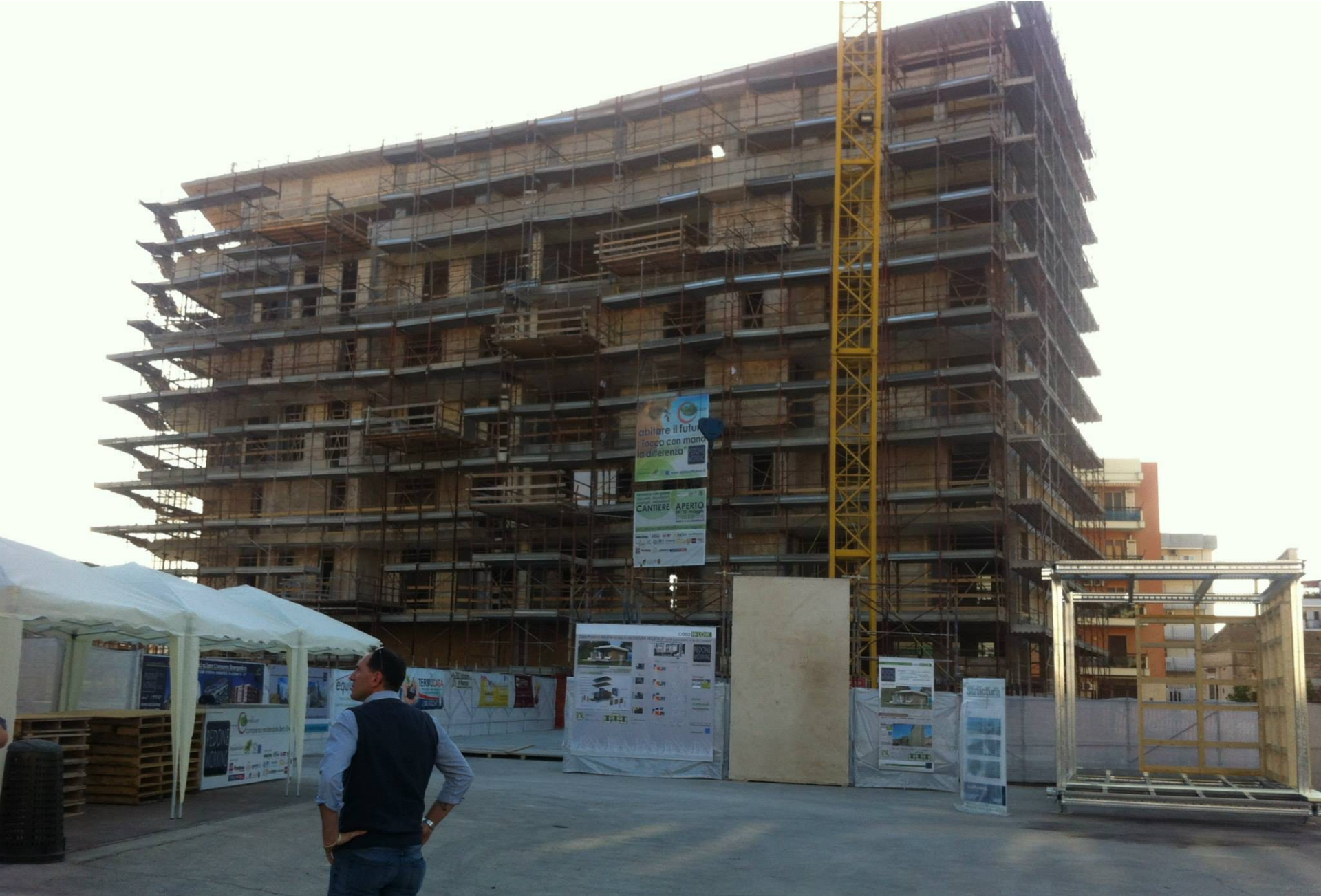
9 floors building in Italy - Equilibrium
