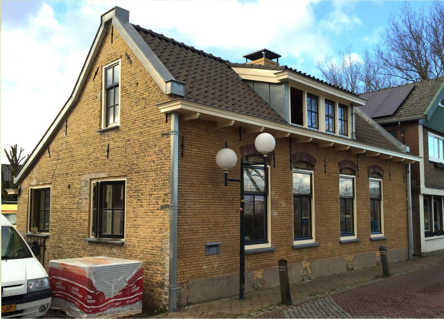
Renovation: Residential house in Zevenhuizen
